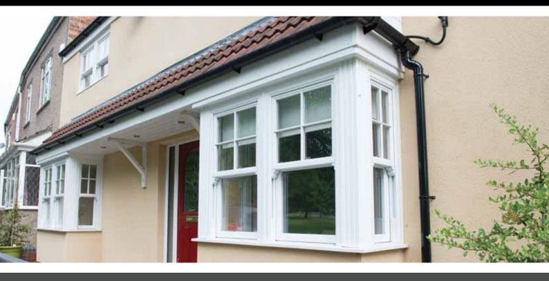
Vertical sliders are suitable for a variety of applications. They are often used in conservation areas and on period properties to replace original timber sliding sash windows. Our PVCu vertical sliders function on a durable spring and spiral balance system. This makes them far more user friendly and less prone to problems than the traditional weights and pulleys system common in heritage sash windows.
